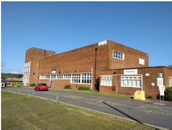
Block 3 Southern and eastern elevations
