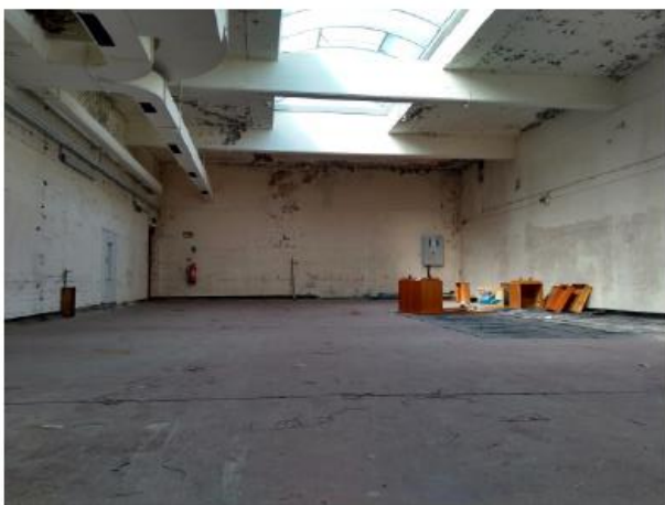
Current internal condition
